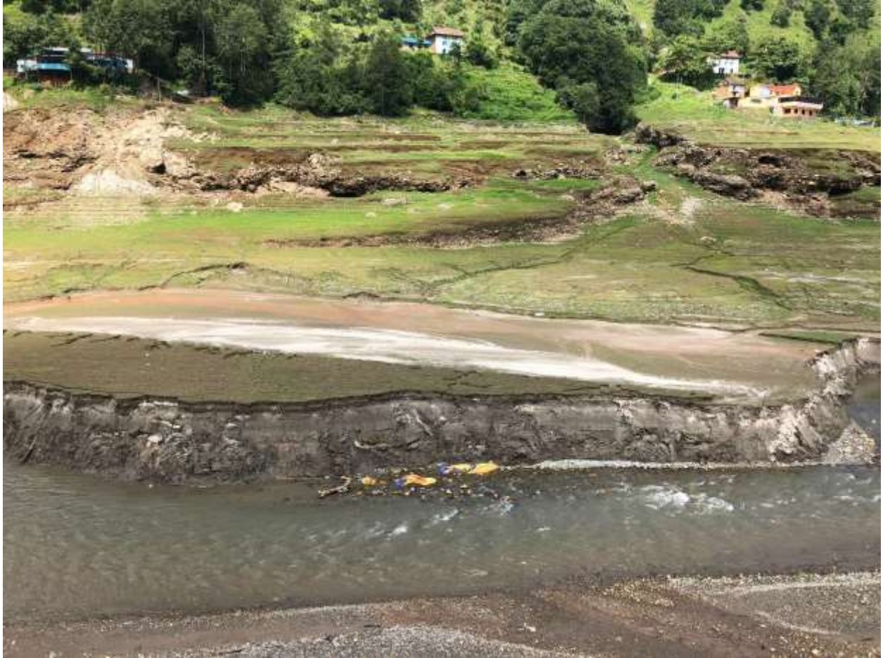
Figure 5: Sand bar deposit on the right bank of Kulekhani reservoir opposite of Chitlang Khola which meets at reservoir
