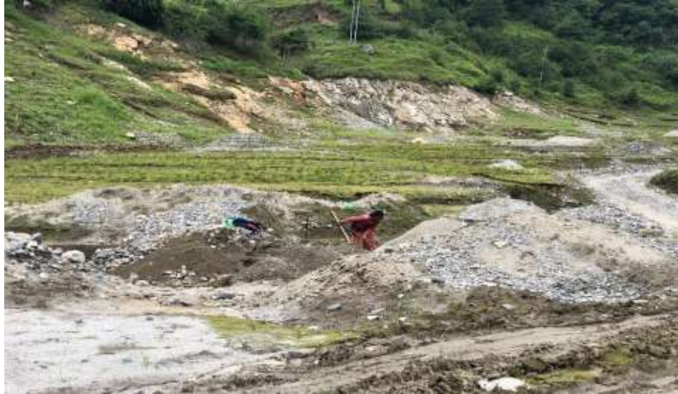
Figure 12: Excavation of deposited materials from the rivers
