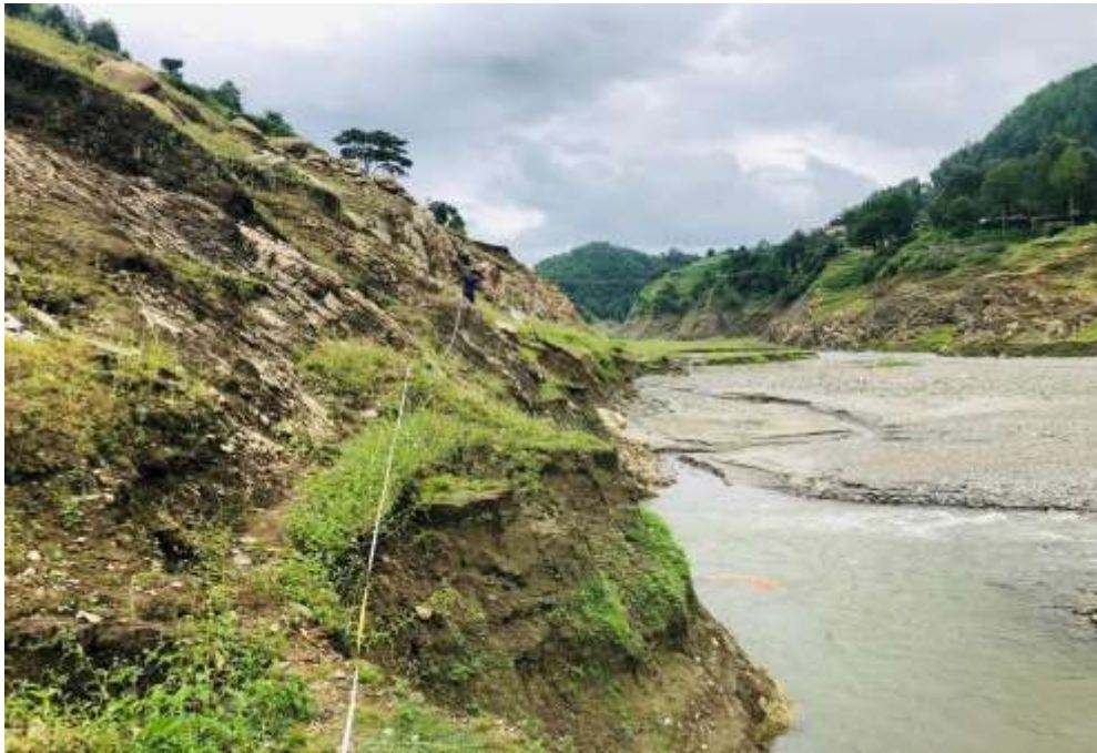
Figure 8: Measurement of slope cutting
