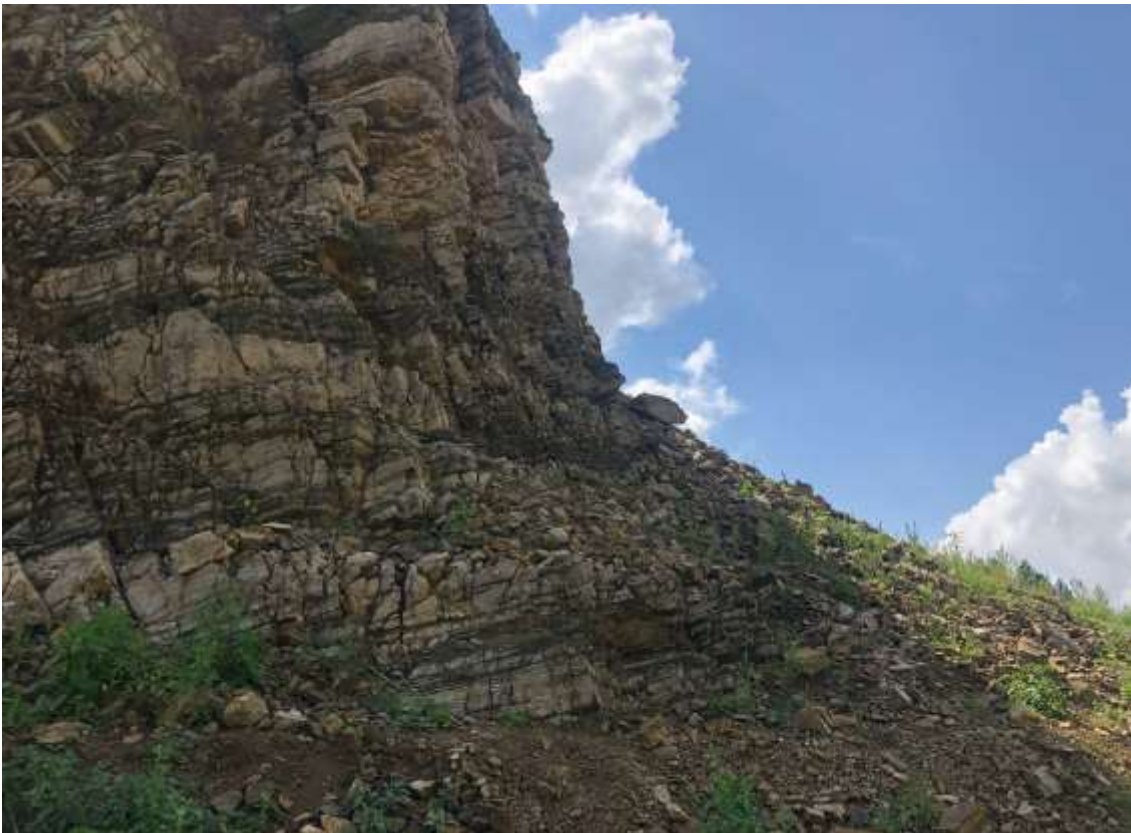
Figure 5: Moderately weathered and highly fractured bedrock on the left bank of Kulekhani reservoir (Wpt: 2463)
