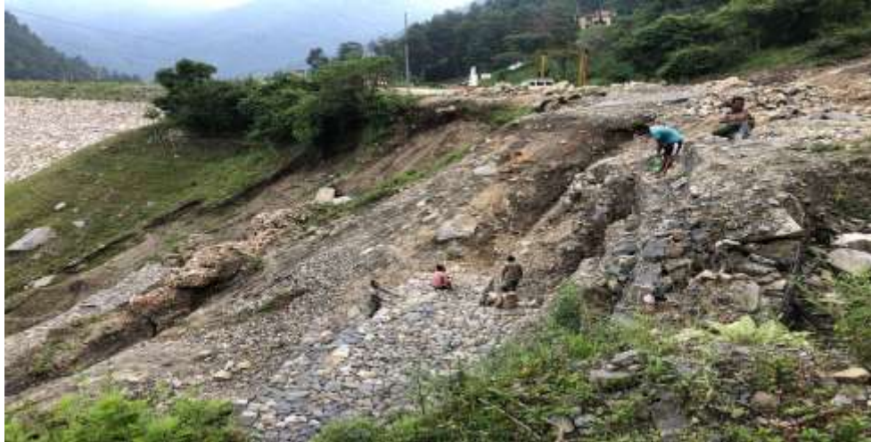
Figure 16: Landslide observed at dam site area
