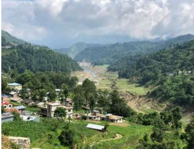
Figure 14: Overview of Kulekhani Reservoir
