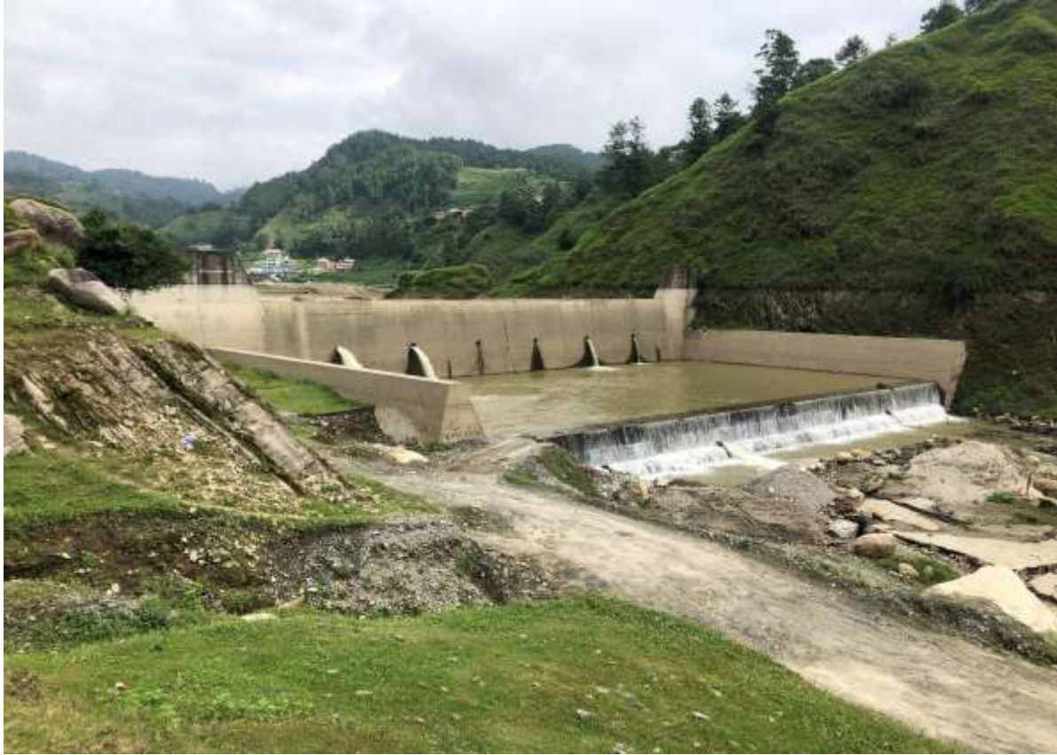
Figure 13: Embankment across the Palung Khola constructed at end section of the Kulekhani reservoir.
