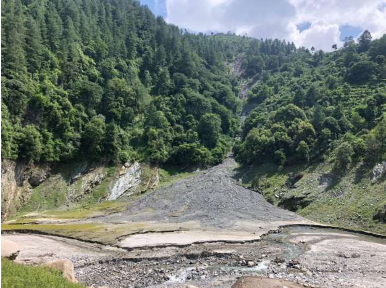
Figure 10: A debris flow occurred due to unmanaged slope after excavation and lack of control measures prior to the failure
