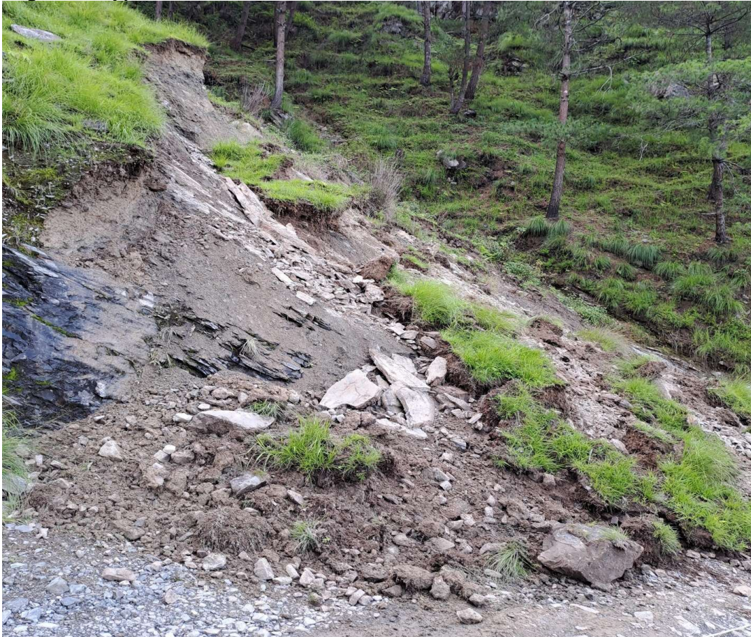
Figure 11 Dhodeni pakha Landslide
