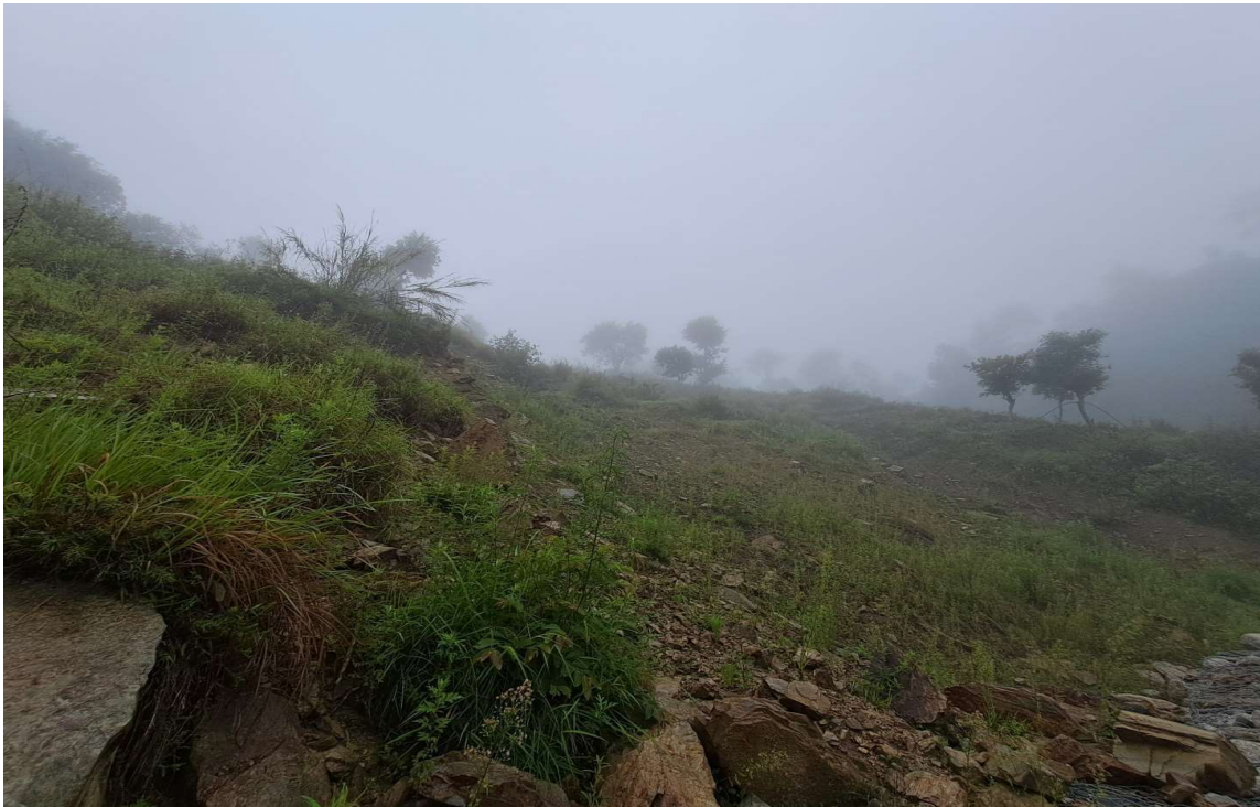
Figure 13 Dhadha gaun 1 Landslide
